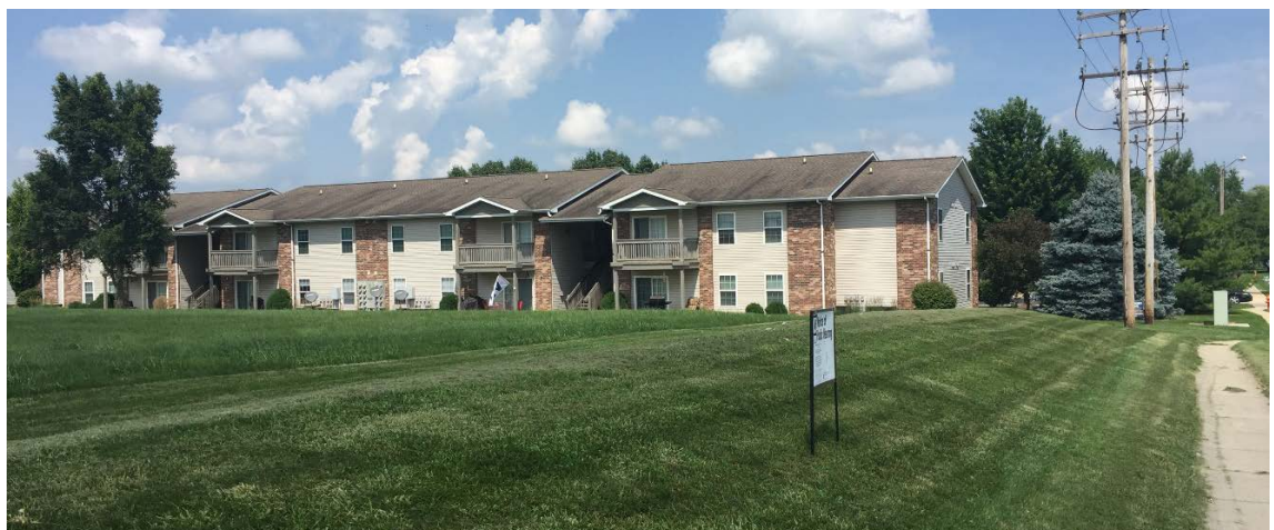
East property line: Stone Ridge Square Apartments
