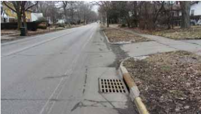
Figure 204 Transverse drainage grate, flush with the pavement, in the Washington Street bike lane east of Vine Street
