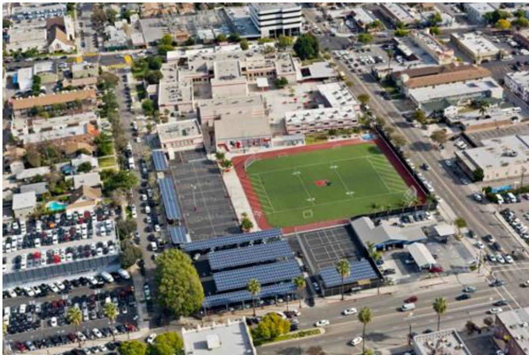
The carport solar installation at the Theodore Roosevelt Middle School in Glendale, Calif. (Source: Borrego Solar)
