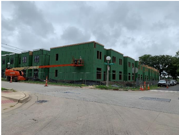
200 Vine townhouse development under construction
