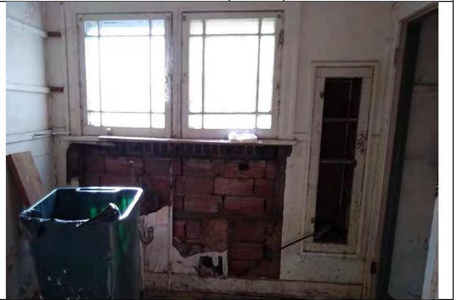
Interior: windows and block wall (A. Fell)
