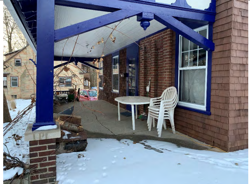
Looking south onto east porch
