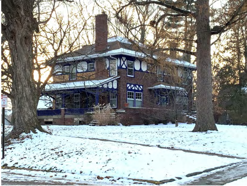
Looking southwest from intersection
