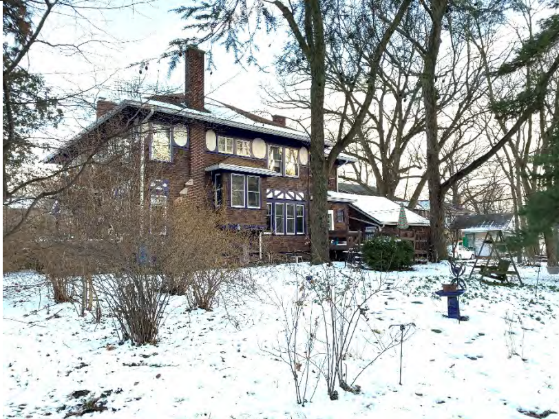
Looking southeast to deck
