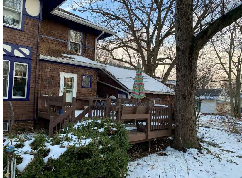
Looking southeast to deck
