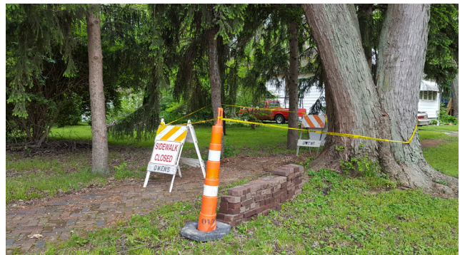
FIGURE 6-12 Brick sidewalk closed for repair on Maple Street in Historic East Urbana
