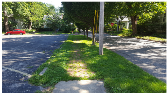
FIGURE 6-13 Brick sidewalk overgrown with grass on Birch Street in West Urbana
