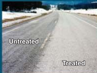
Residential street application.
