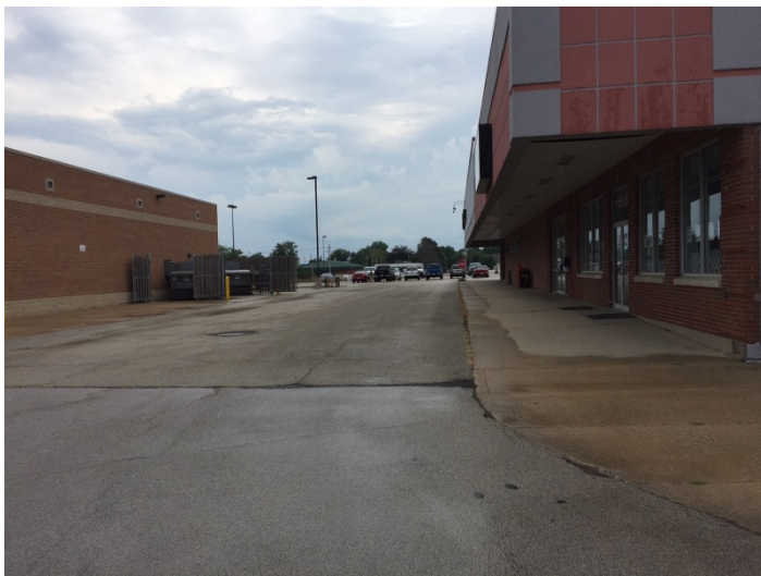
Figure 5. Storefront sidewalk facing south.
