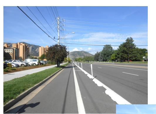
Overbuilt 6-lane roadway converted to 4-lanes w/ protected cycle track.
