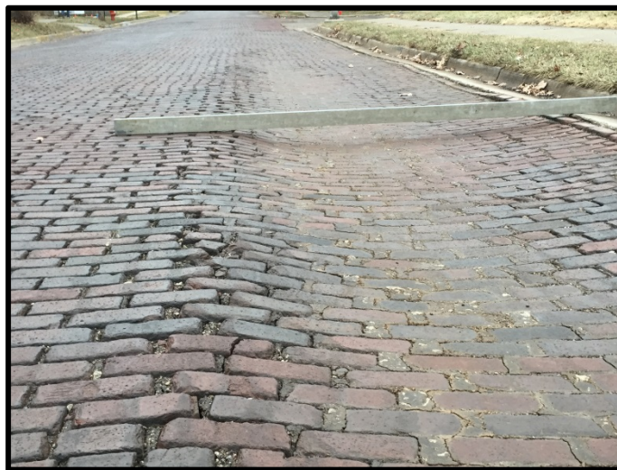
Photo 2: High Severity Rutting
