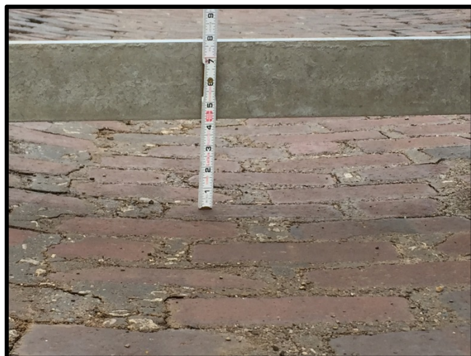
Photo 3: Rutting Depth \pm 4.5''
