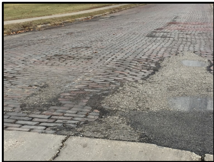
Photo 1: Asphalt Patch Used To Correct Rutting
