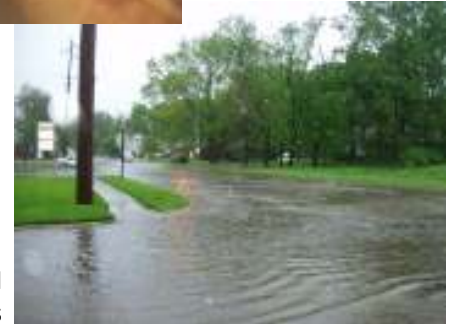
Street Flooding from Clogged or Undersized Storm Sewers
