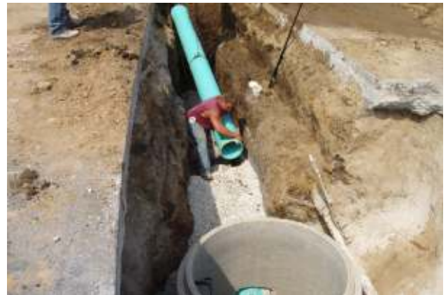
Broadway Avenue Storm Sewer Replacement
