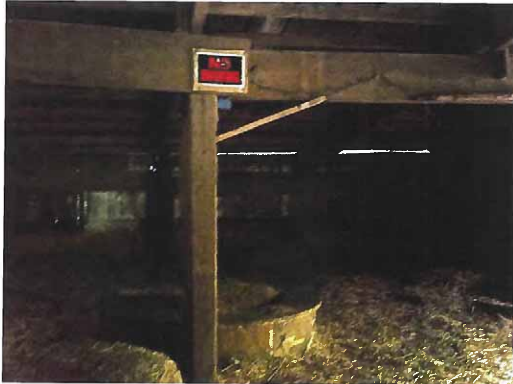
East Barn interior
